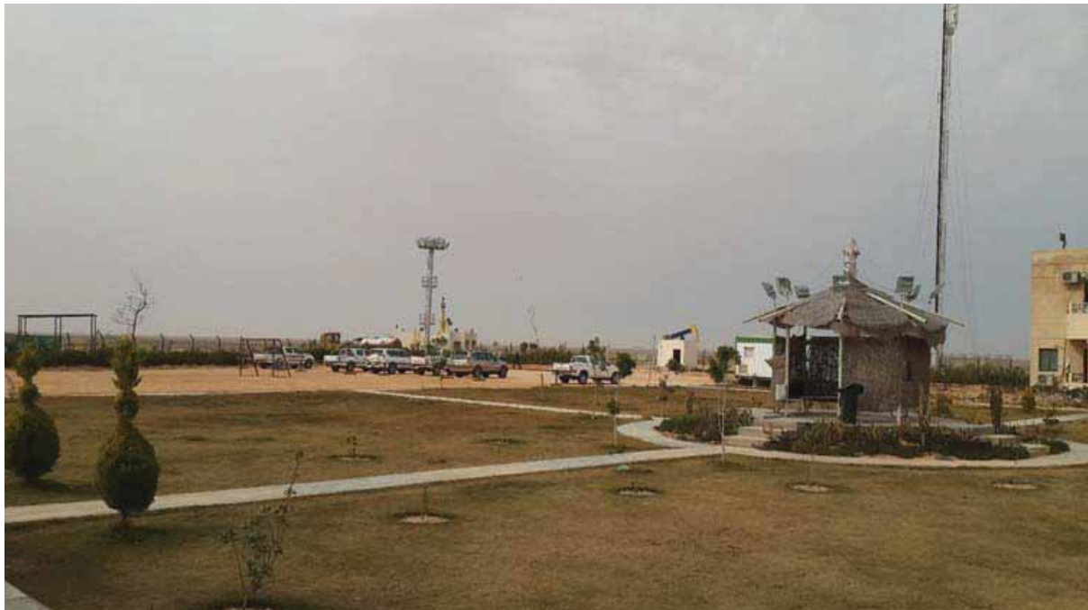
Figure AIII.9: Main Site Office, Carpark and Fencing
