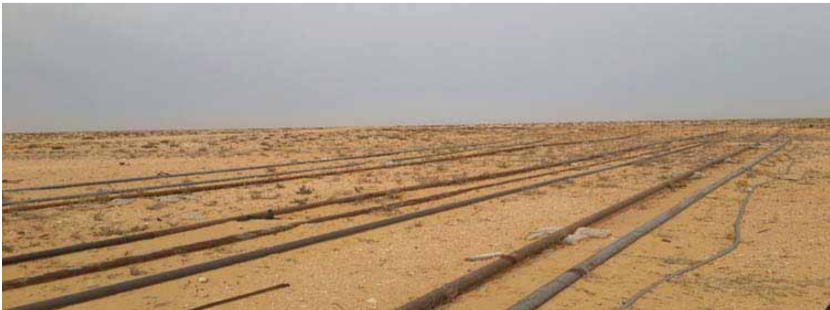
Figure AIII.3: Pipeline Installation
