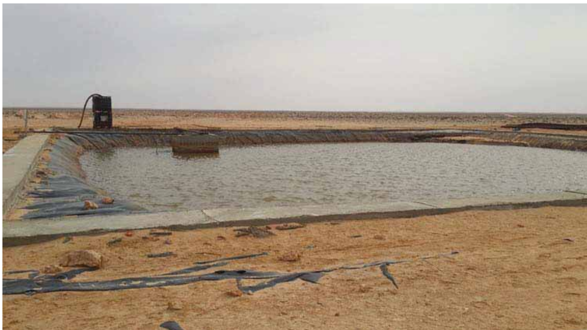
Figure AIII.8: Produced Water Lagoon
