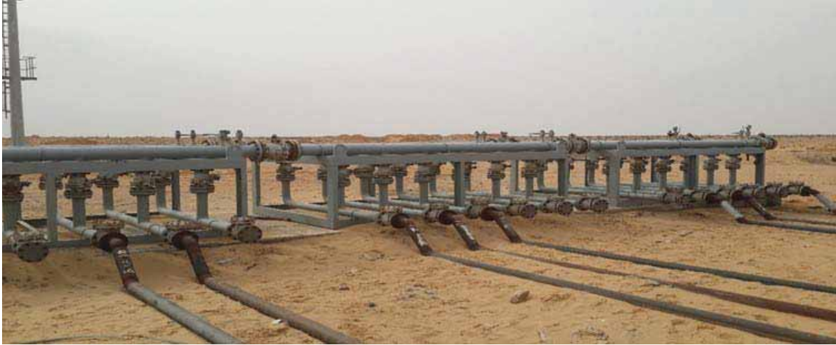
Figure AIII.2: Manifold
