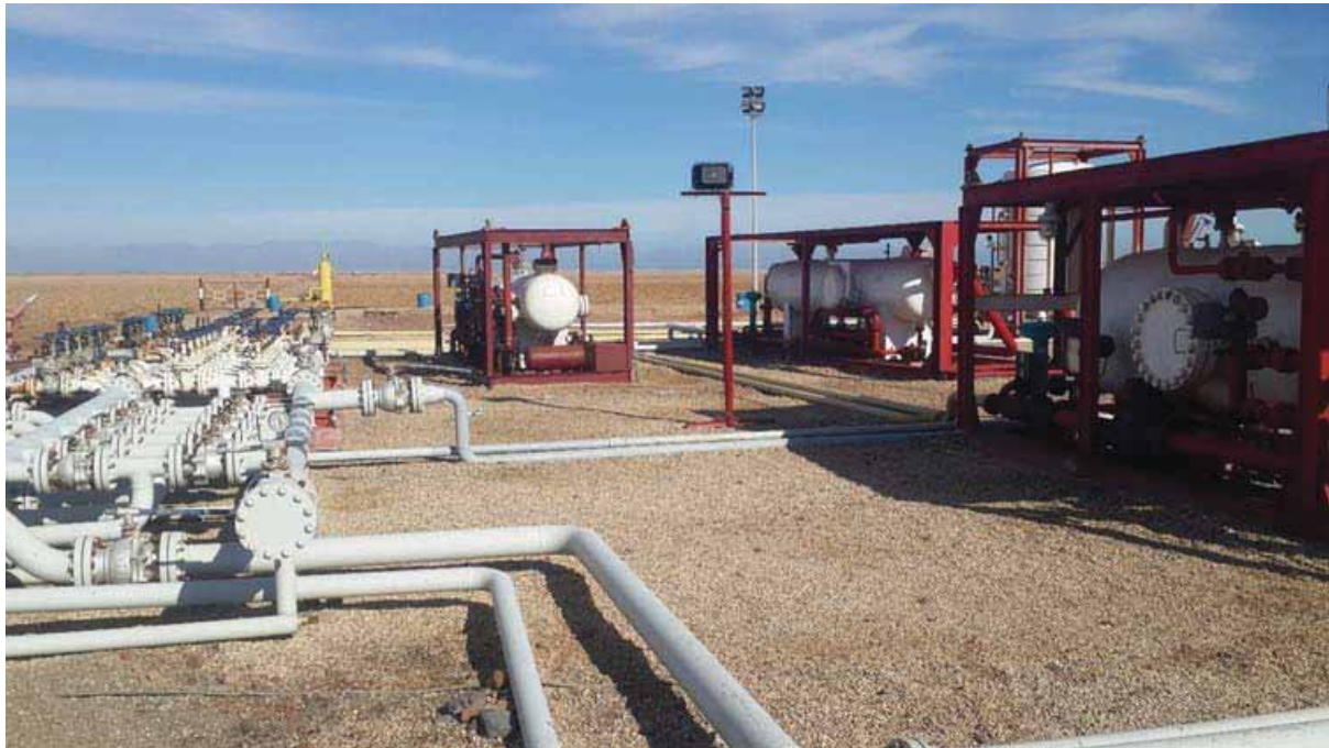
Figure AIII.21: Three-Phase Separator Unit
